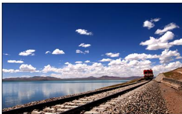
The newly built Gormo-Lhasa Railway
