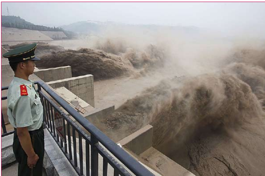
Water rushes through the Xiaolangdi Dam on the Yellow River in central China's Henan province. Officials released the water to clear sediment in an attempt to prevent summer flooding. (Photo credit: STR/AFP/Getty Images)
