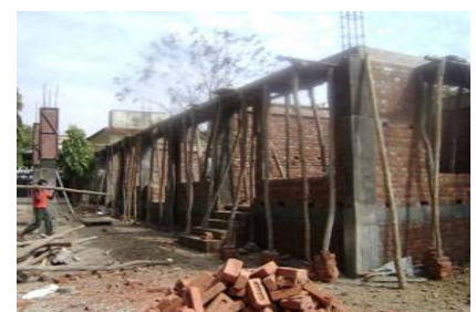
View of LTA Office, Dekyiling under construction
