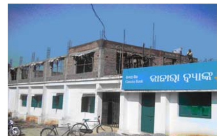
View of LTA Office, Orissa under construction
